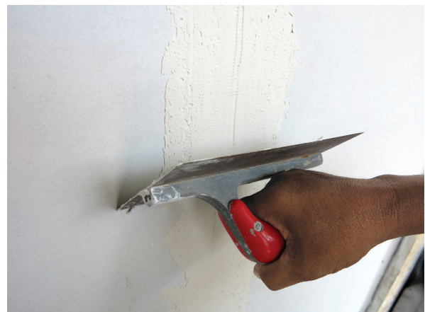
Apply subsequent covering of plaster compound to finish
