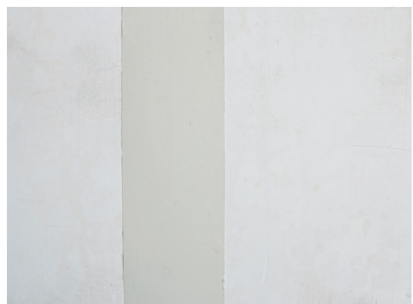
Final joint after finishing with trowel
