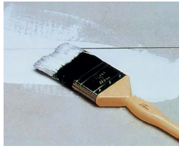
Preparing joint with primer
