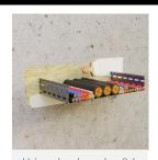
Using a brush, apply a 0.6 mm thick layer of **PiroCoating** on the wool over a length of min. 50 mm from the cable tray
