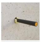
Fill the space between the cable and the partition tightly. Use mineral wool with a density of min. 50 kg/m<sup>3</sup> or cement mortar
