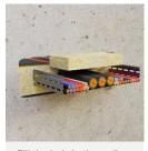
Fill the hole in the wall on both sides with mineral wool boards with a minimum density of 50 kg/m<sup>3</sup> and a maximum thickness of 40 mm
