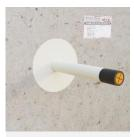
Mark the penetration with the attached label, mark **PiroCoating** on it, enter the date and name
