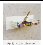
Appy on the cables and cable tray a layer of fireproof **PiroCoating** with a brush. Coating with a brush. Coating with a thickness of min. 1.2 mm on the length of min. 300 mm from the partition
