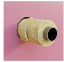
Fill the space between the pipe insulation and the partition tightly. Use mineral wool with a density of min. 60 kg/m<sup>3</sup>
